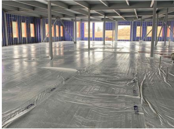
Preparation for slab on grade pour in the classroom wings (04/22/2022)
