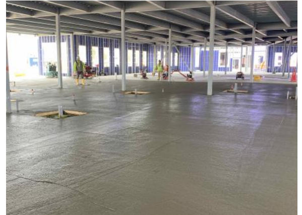
Completed slab on grade pour in the classroom wing (04/28/2022)
