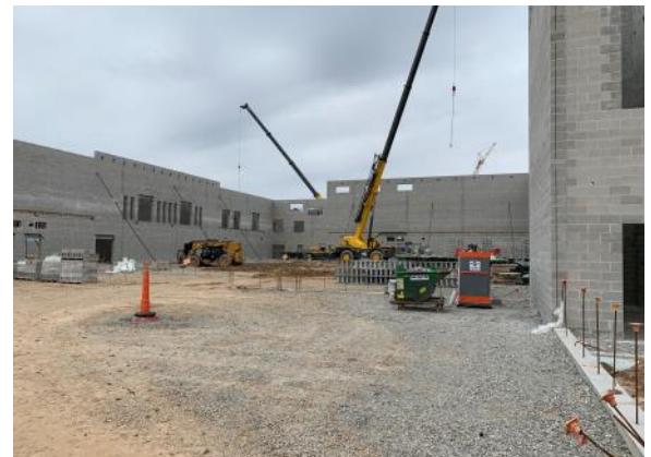
Masonry walls going up in the competition gym (04/12/2022)
