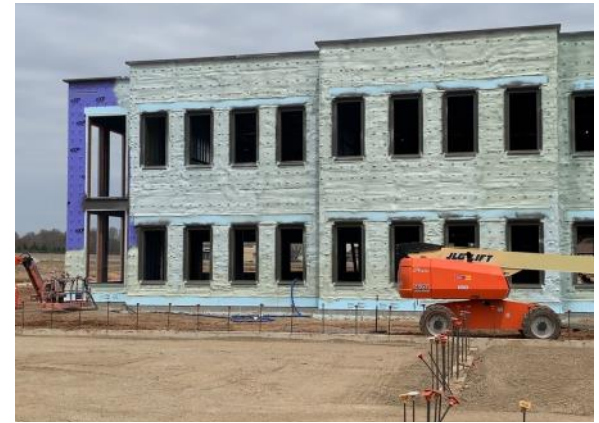
Exterior spray foam installation on the Westmost classroom (04/29/2022)
