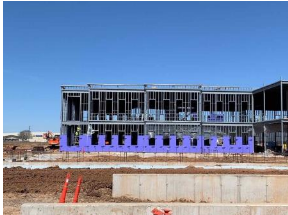
Exterior steel stud framing and sheathing on the West classroom wings (04/11/2022)
