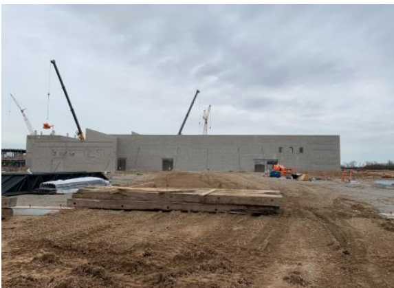
Looking South at the wrestling room and auxiliary gym (04/12/2022)
