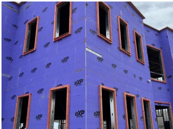
Exterior steel stud framing and sheathing on the West classroom wings (04/11/2022)
