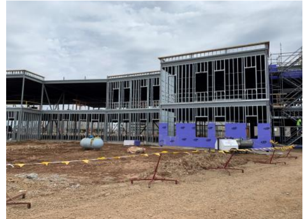
Northwest classroom wing exterior steel stud framing (04/11/2022)
